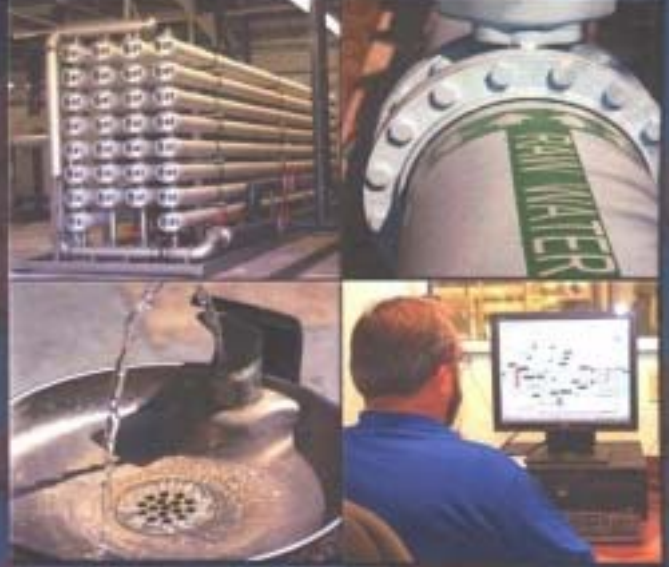
REVERSE OSMOSIS WATER TREATMENT PLANT
