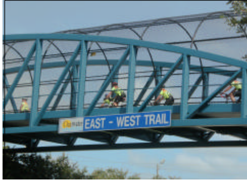
McMullen Booth Overpass
