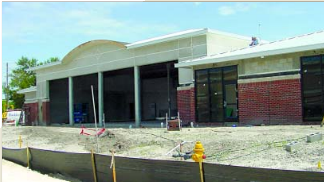
Construction is two-thirds complete on the new Clearwater Mall Fire Station.
