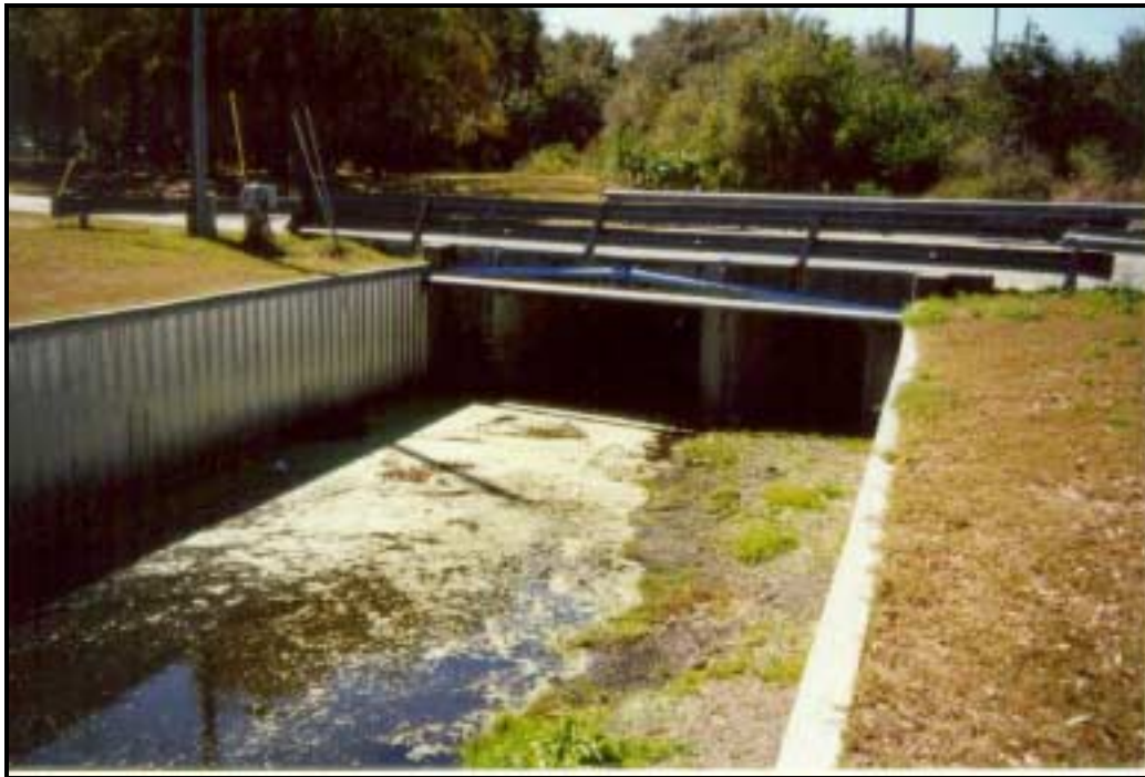
Figure 2.1-7 Box Culverts Downstream of King's Highway Monitoring Station
