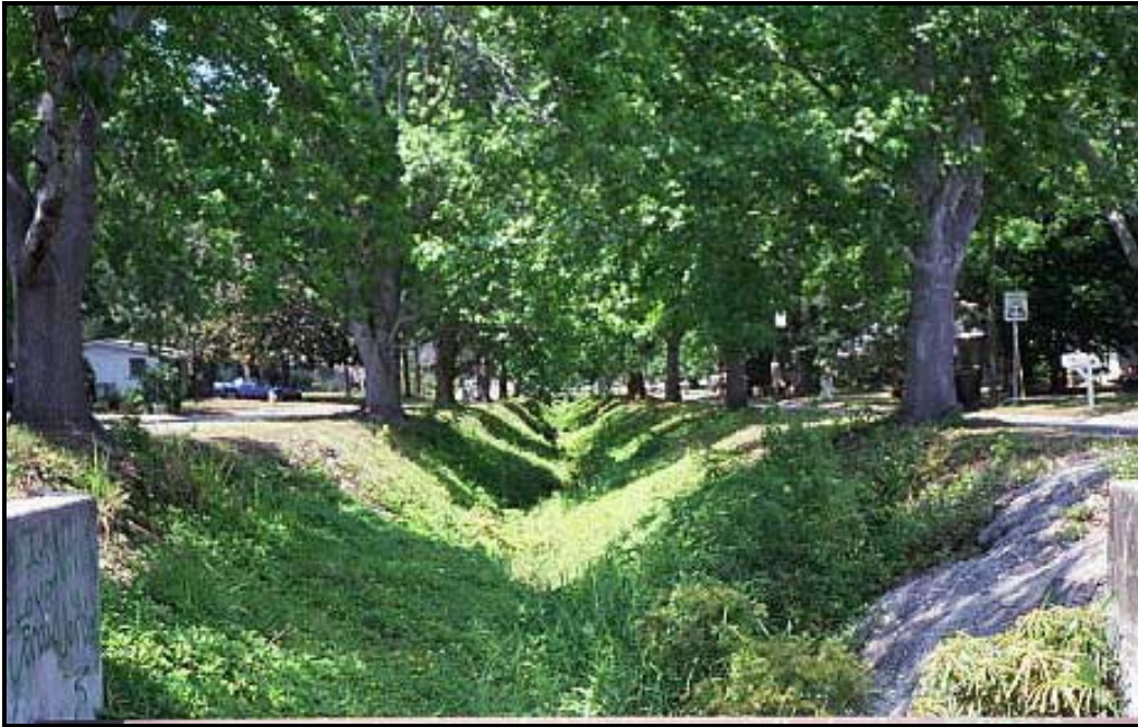
Figure 3.1-19. Stevenson Creek Channel and Trees Along Hillcrest Avenue, Between Jeffords Street and Browning Street (to remain)
